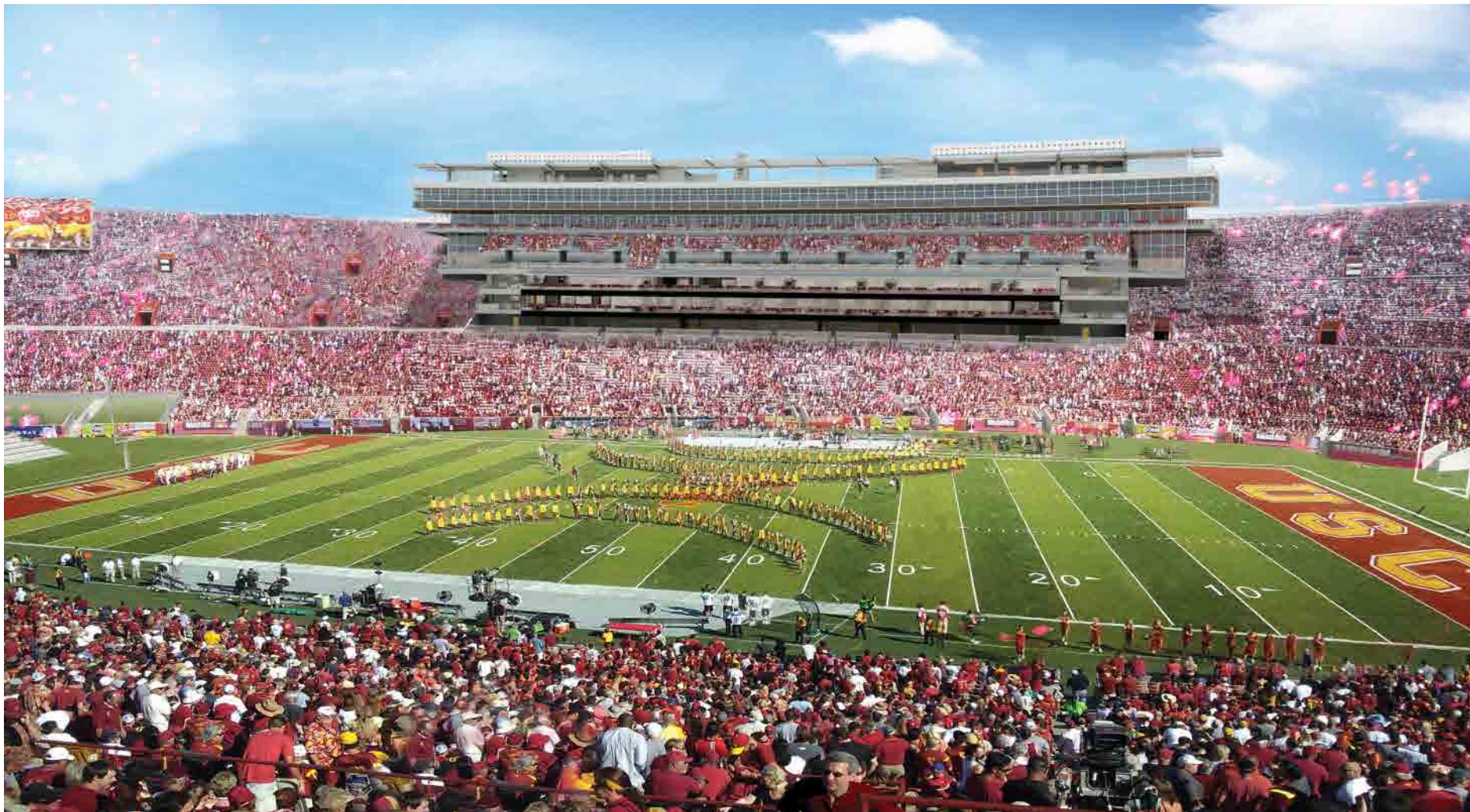
Field side view of the new South Stadium addition
