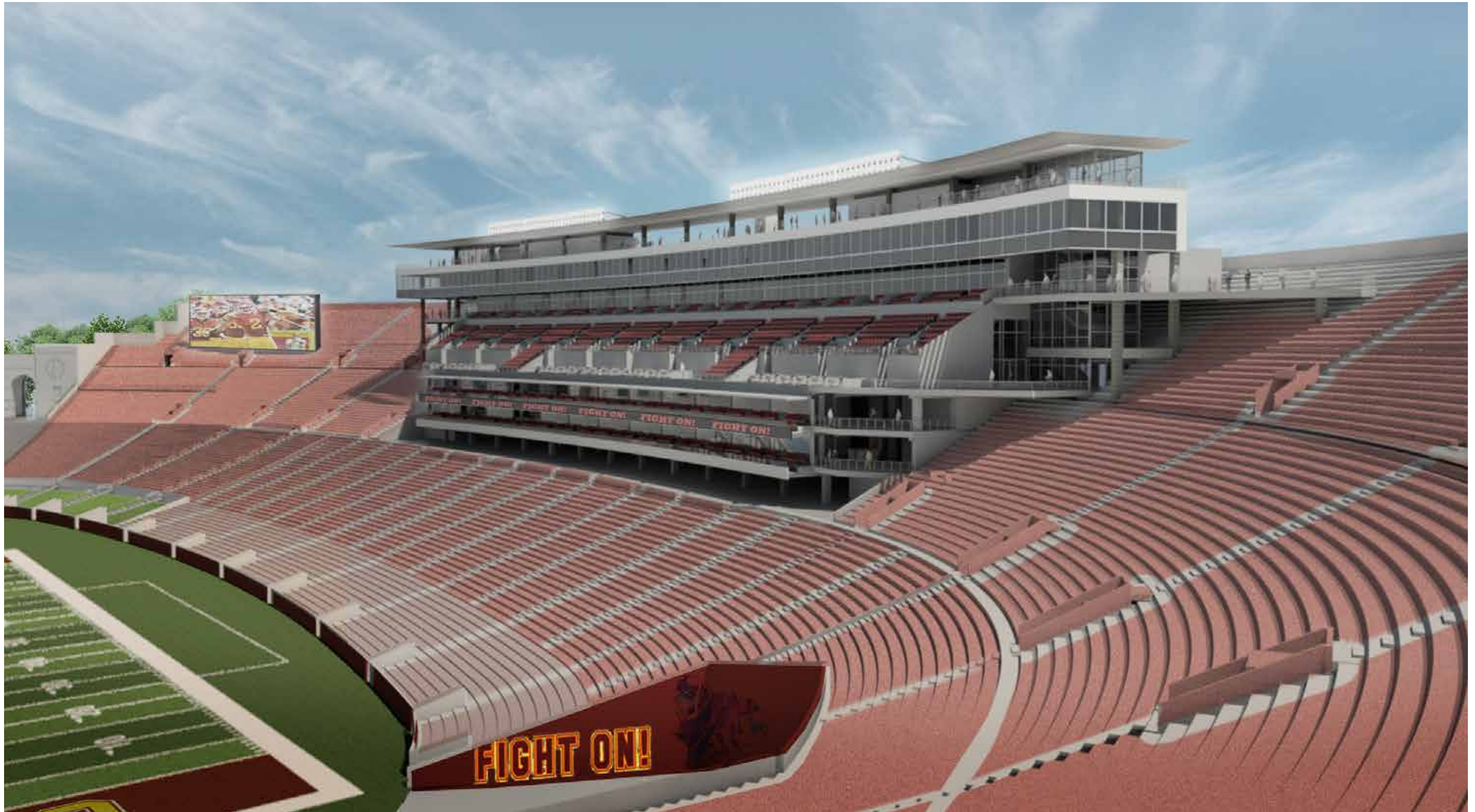
South Tower, View looking Southeast Seats have been added in the areas adjacent to the addition.
